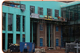
Installing Brick on Front
