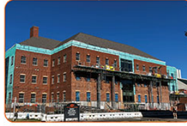
Finishing Brick on South Side
