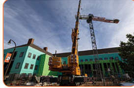
Removing Crane
