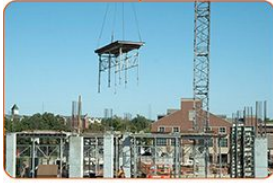
Installing Forms for Concrete
