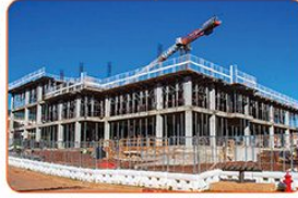
Constructing Three Floors
