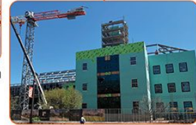
Installing Windows &amp; Roof
